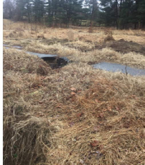
Figure 7: Looking Along the Path of a Dilapidated Storm Sewer Pipe
