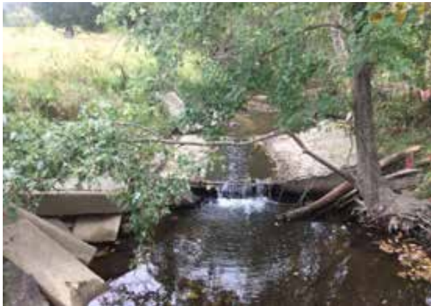
Figure 5: Existing Concrete Pedestrian Bridge that has Collapsed
